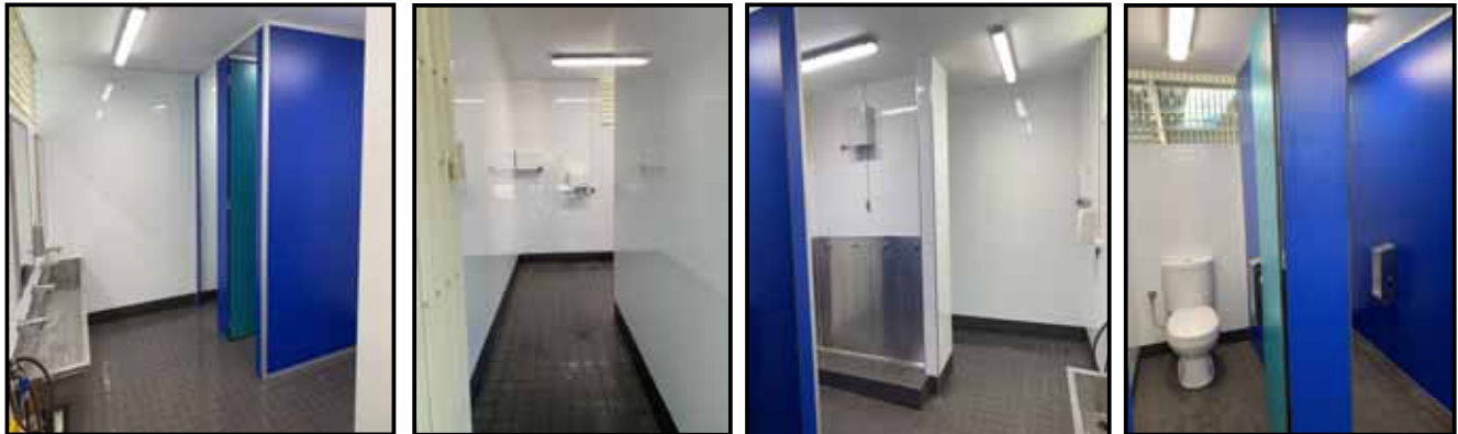
Boy's toilets – wash basins, entry corridor & toilet cubicles.
