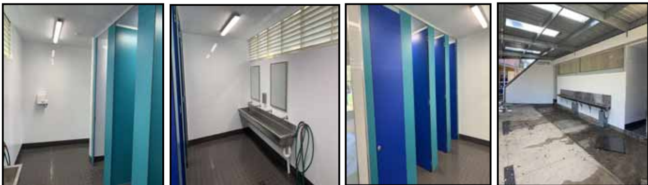
Girl's toilets – general area & floors, wash basins & mirrors, partitions & outside entry area
